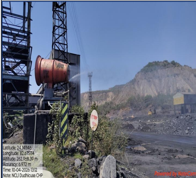
Fig:- Anti-Smog Gun Sprinkling in CHP
