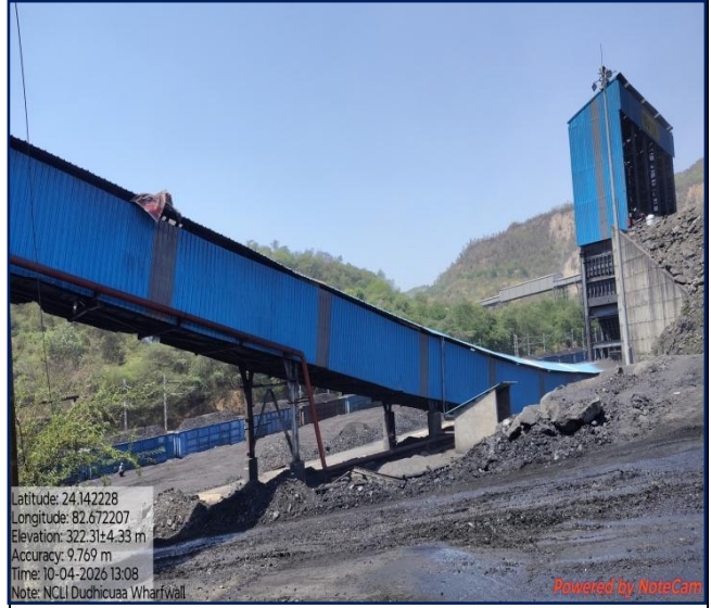
Fig:- Transportation of Coal through Covered Conveyer Belts
