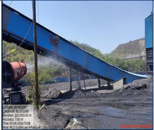
Fig:- Anti-Smog Gun Sprinkling in Wharf Wall
